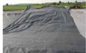
The panels are available in numerous sizes which can be selected to accommodate the dimensions of the project. This reduces losses and limits the cutting and field seaming. The list of available Firestone GeoGard EPDM panel sizes is included in the Technical Information Sheet (TIS) on page 9.
