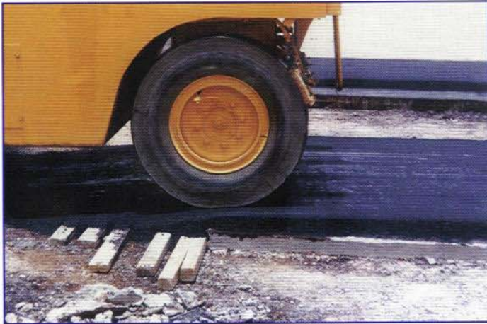
Asphalting directly on FIBREPOL
